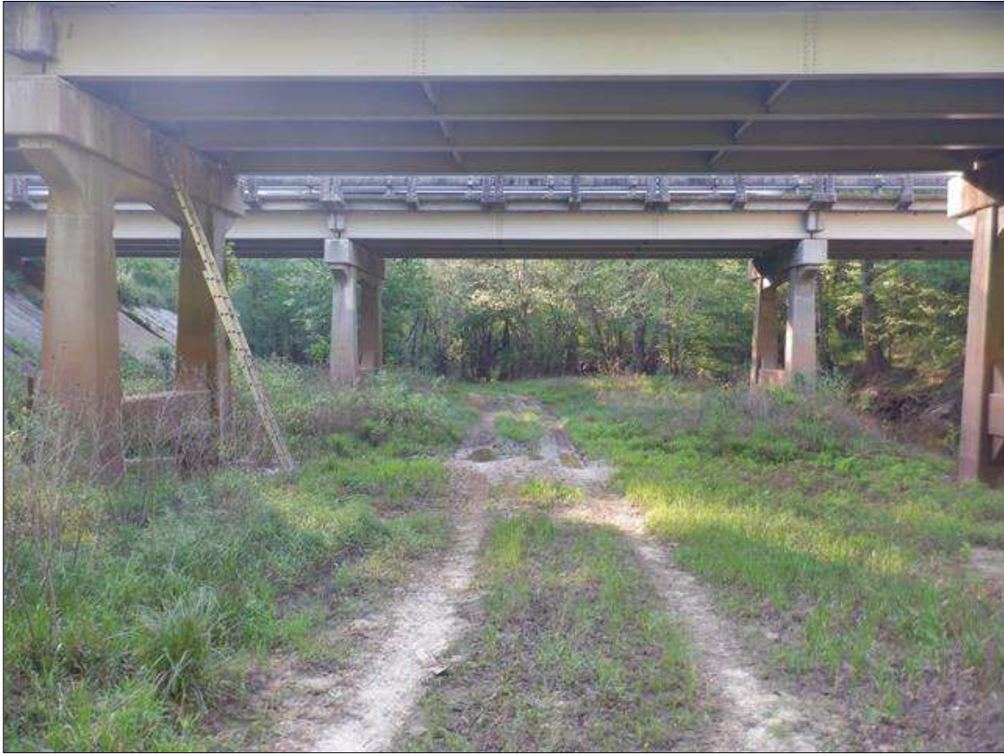
SPAN 3 CLEARANCE OPENING, GREENWAY, LOOKING EAST
