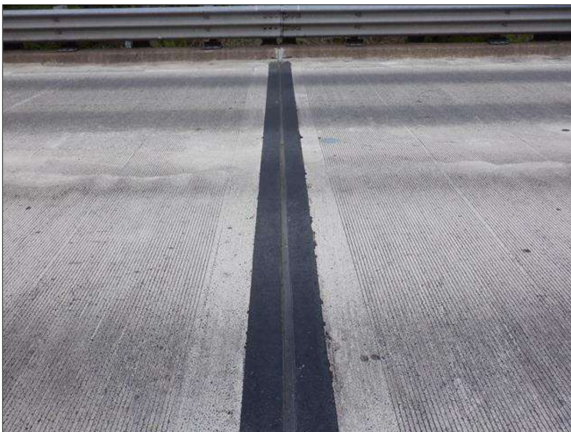
JOINT OVER BENT 2 LOOKING WEST
