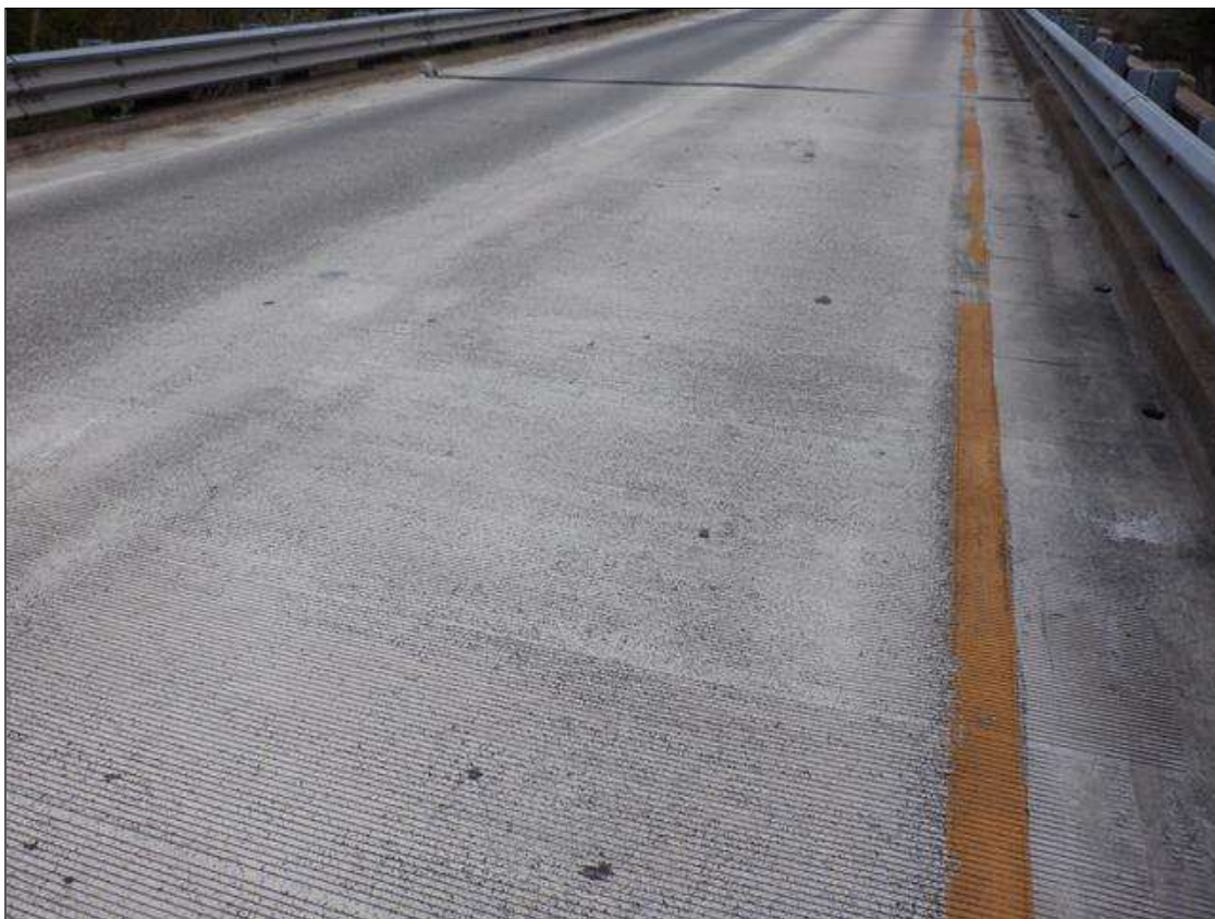
SPAN 1 CONCRETE WEARING SURFACE LOOKING NORTH
