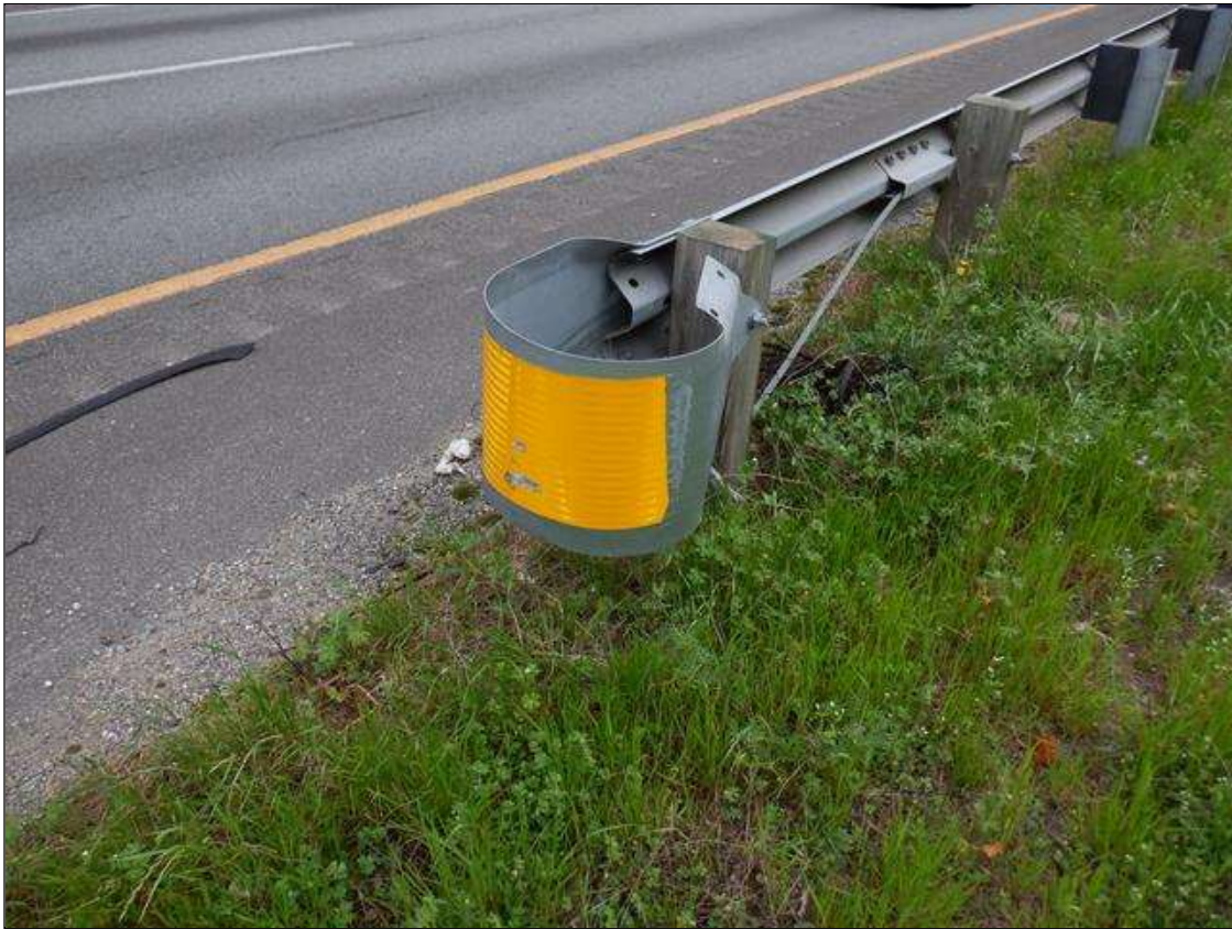
SOUTHEAST GUARDRAIL TERMINAL (SOUTHWEST SIMILAR)
