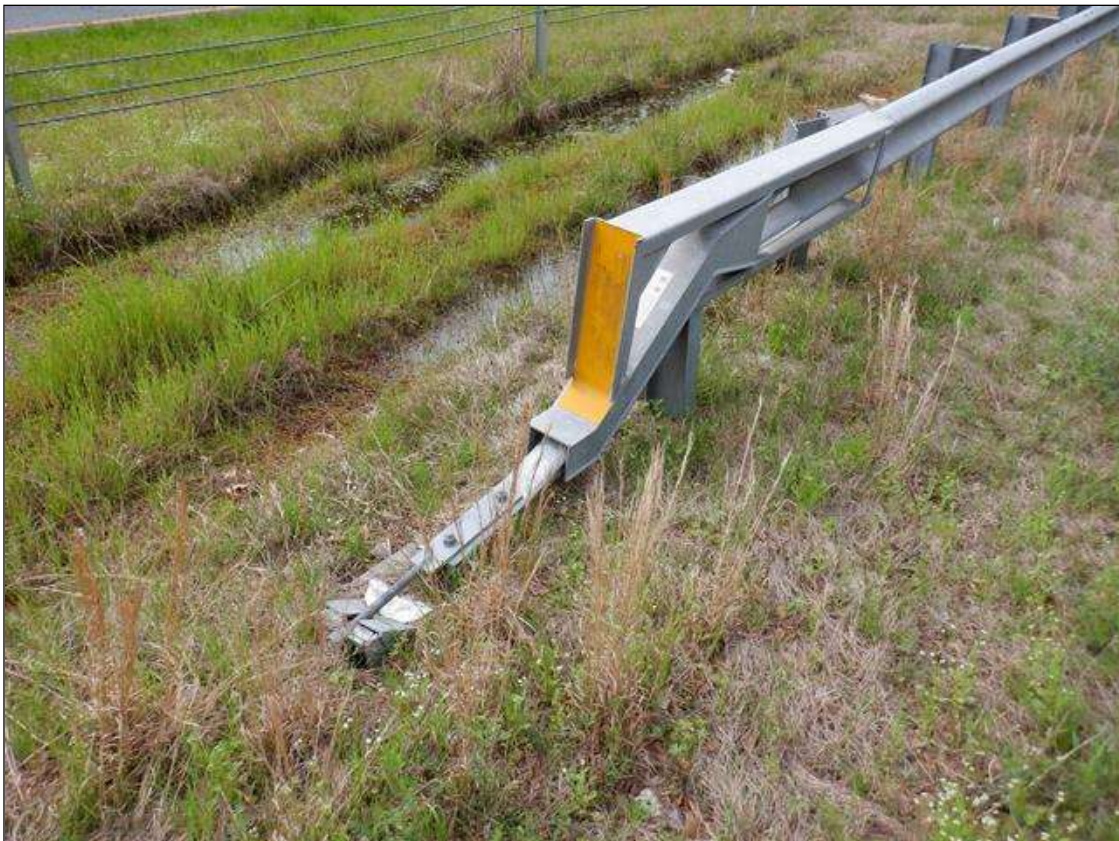
NORTHEAST GUARDRAIL TERMINAL (NORTHWEST SIMILAR)
