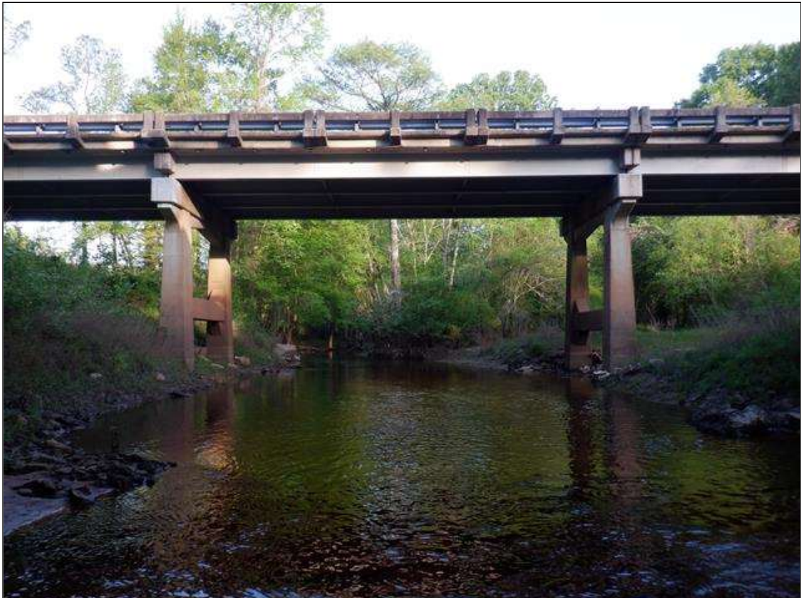
SPAN 2 WATERWAY OPENING LOOKING WEST
