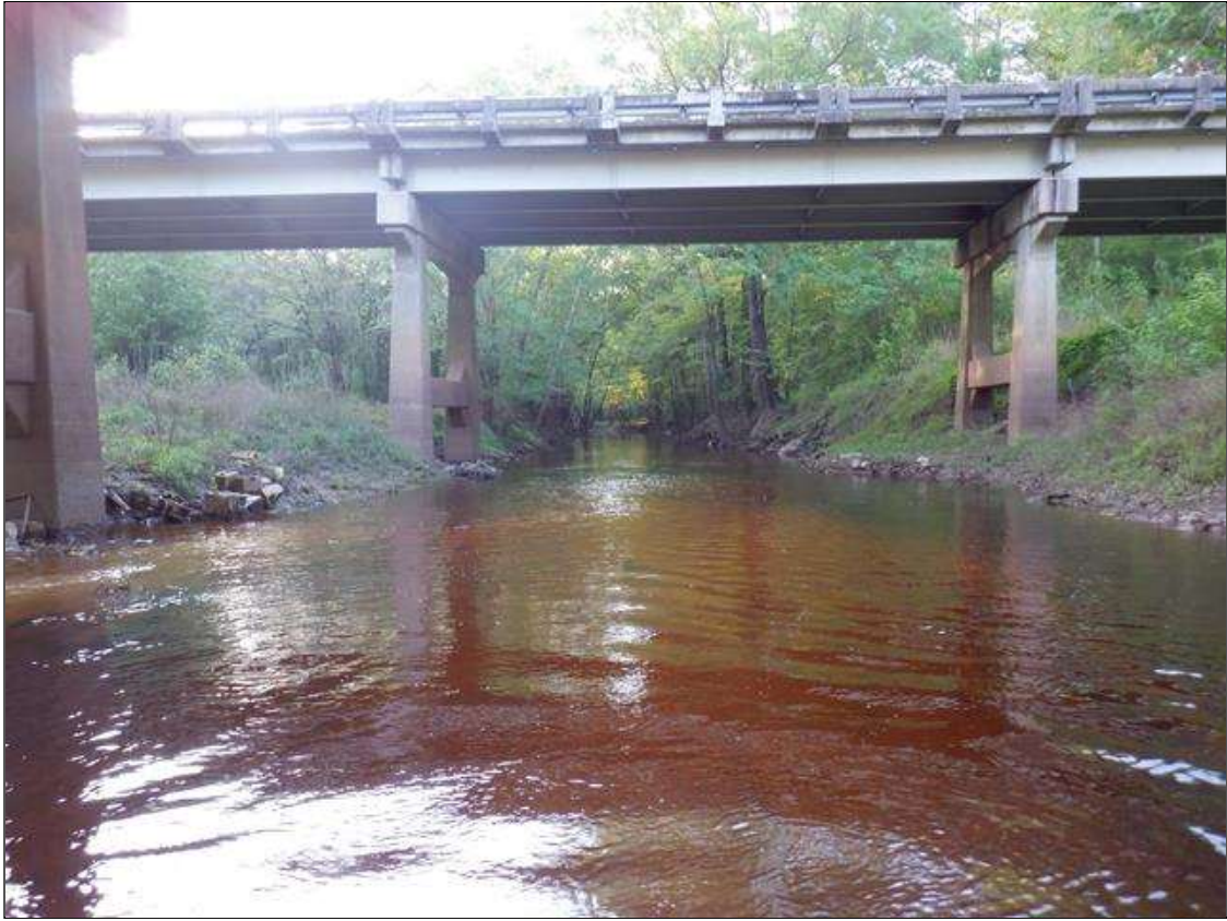
DOWNSTREAM VIEW LOOKING EAST
