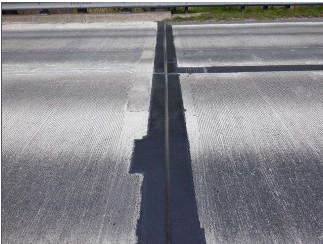
JOINT OVER END BENT 2 LOOKING WEST
