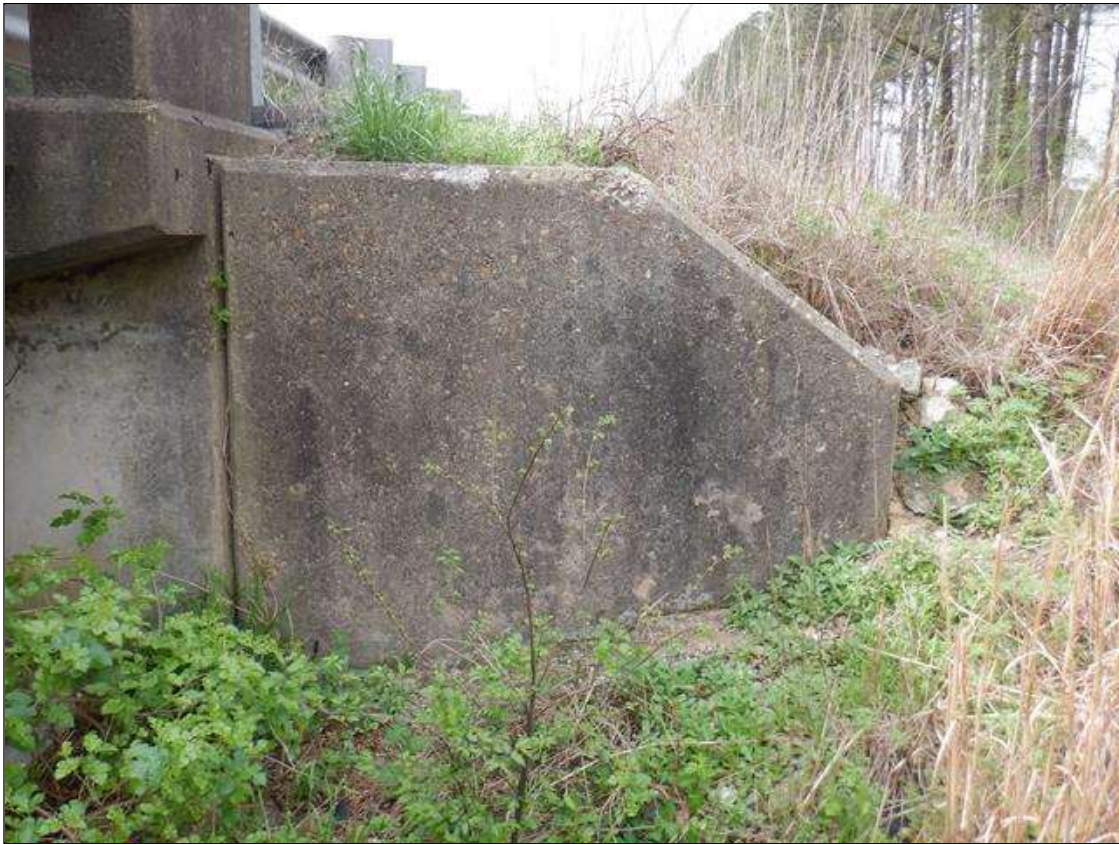
SOUTHWEST WINGWALL (OTHERS SIMILAR)
