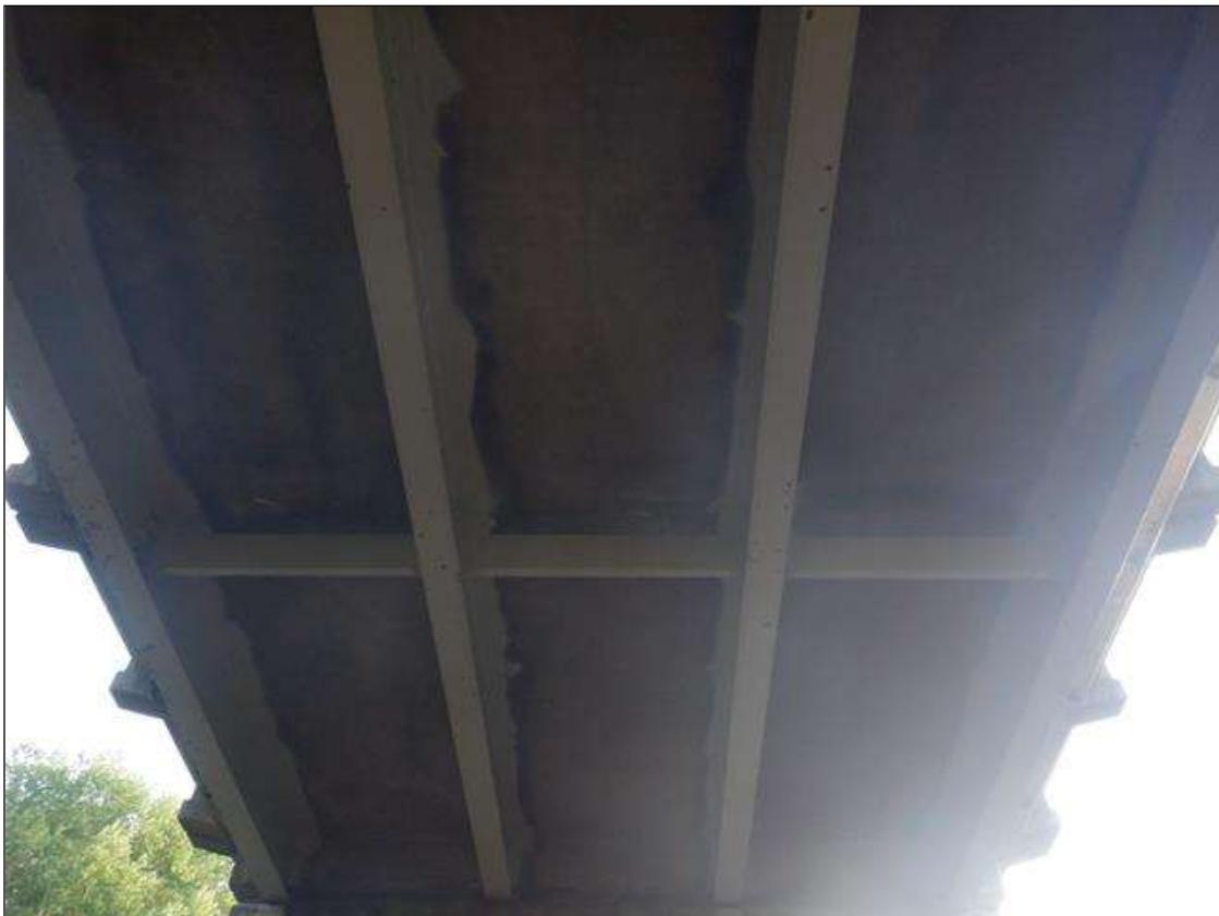
SPAN 2 SUPERSTRUCTURE UNDERSIDE LOOKING NORTH
