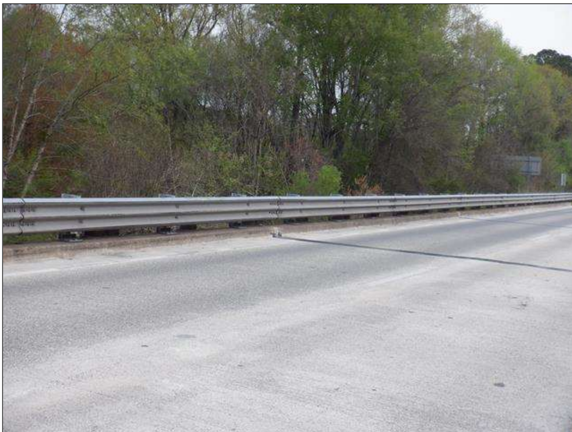
WEST BRIDGE RAIL
