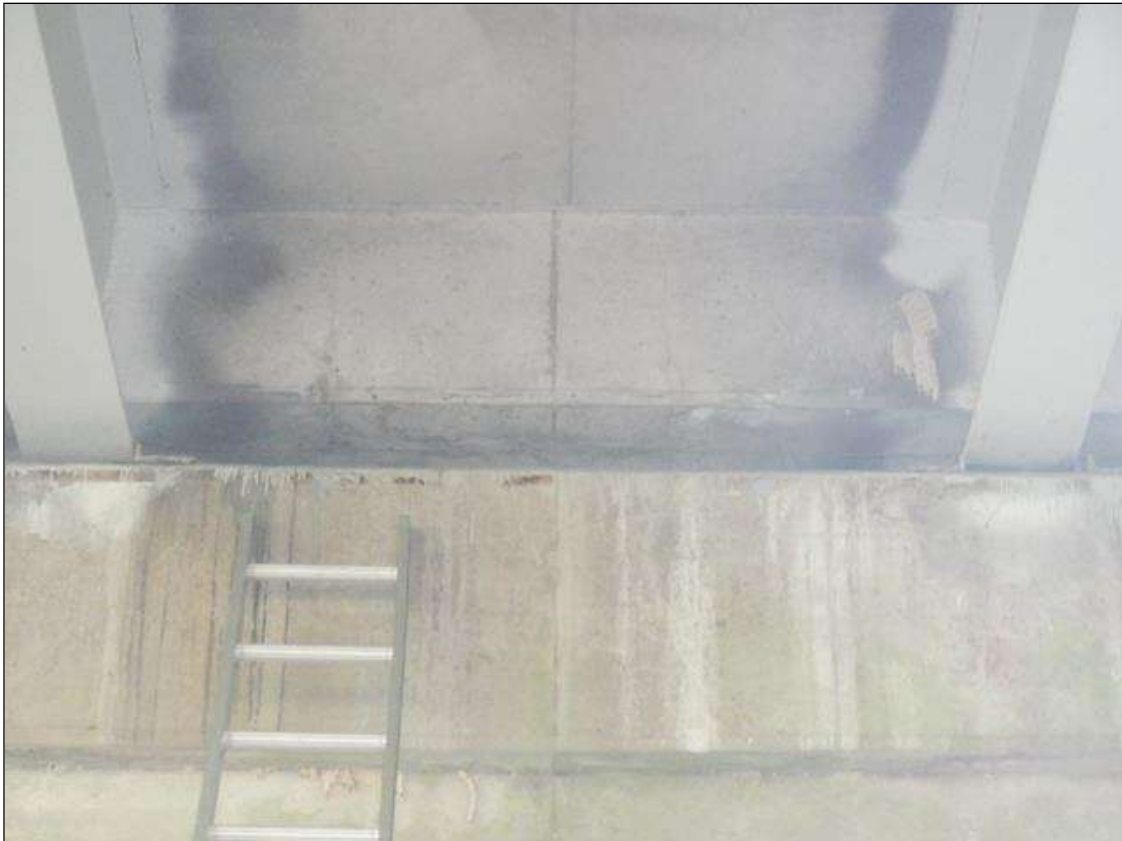
BENT 3 BAY 2 DIAPHRAGM LOOKING NORTH (OTHERS SIMILAR)
